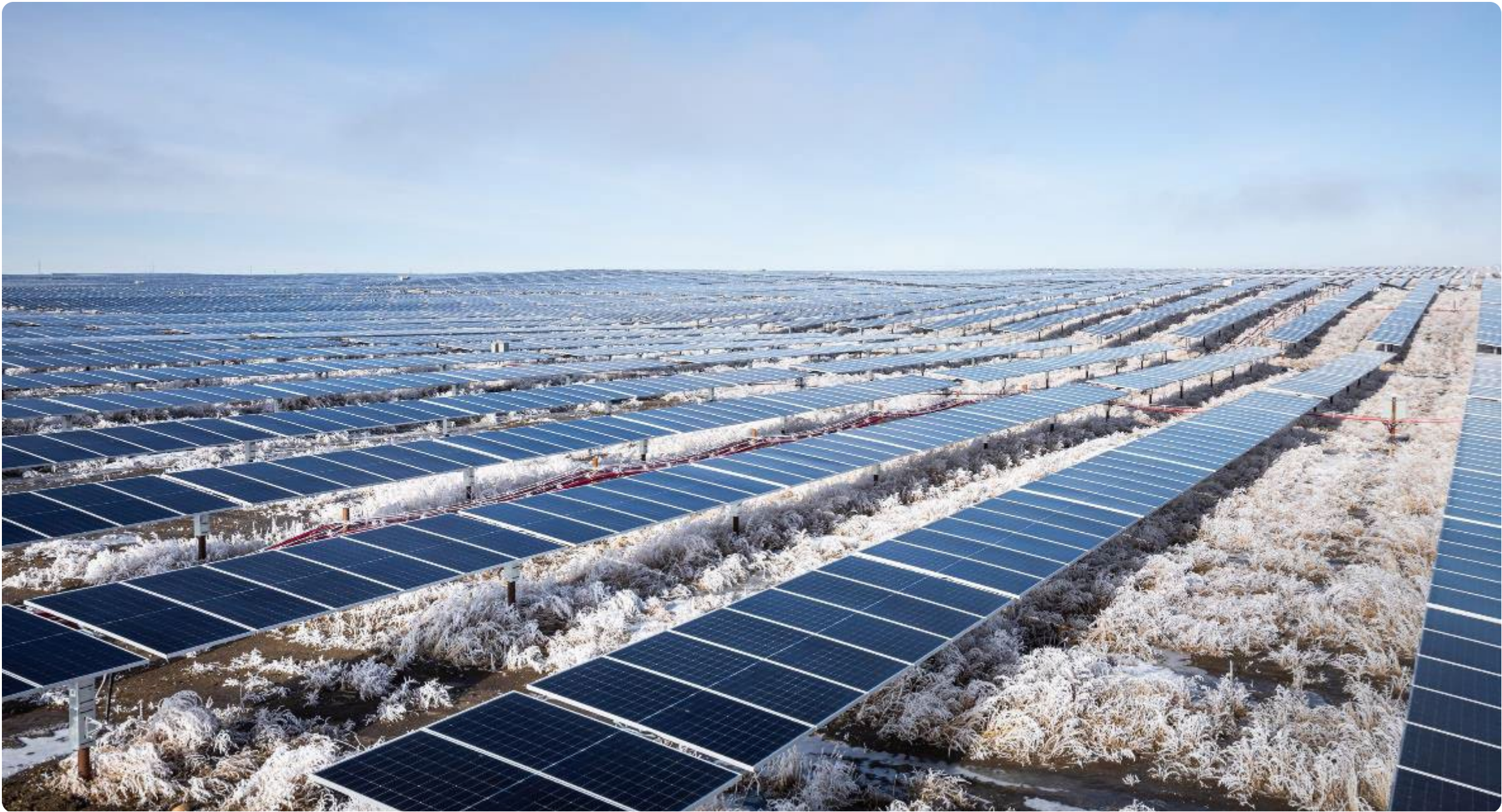
Travers Solar Project, Alberta
