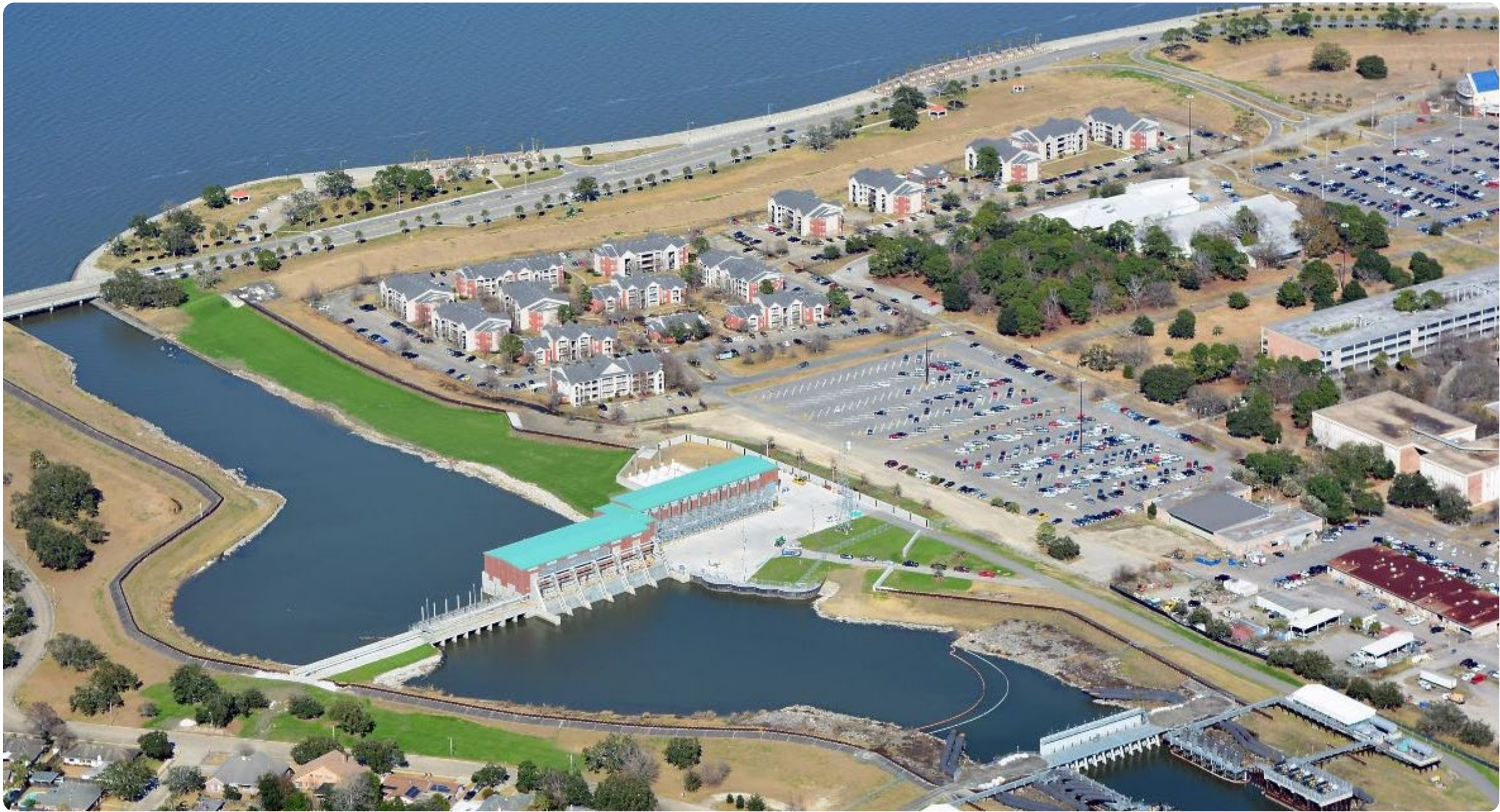
New Orleans Permanent Canal Closures and Pumps Project
