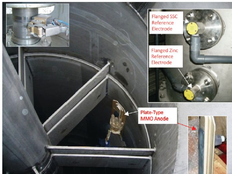
FIGURE 3 Plate-type MMO anode and flanged reference electrodes.
